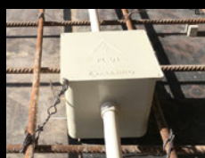
Custom conduit holes for perfect fit
